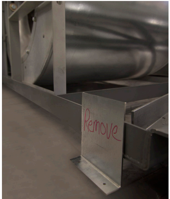
FIGURE 7: TYPICAL FAN BASE SHIPPING BRACKET ▼
