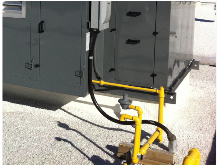
FIGURE 16: ELECTRICAL INSTALLATION W/PITCH POCKET ▼
