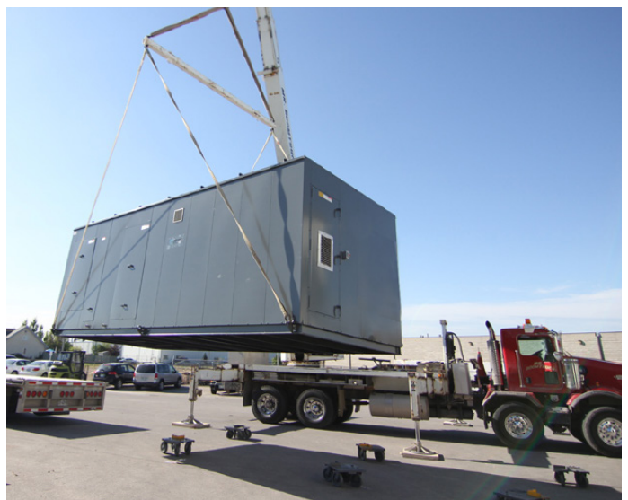
FIGURE 6: TYPICAL SPREADER BAR ARRANGEMENT ▼
