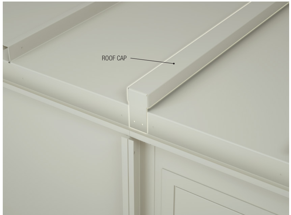
FIGURE 6: ROOF CAP INSTALLED TO COVER JOINTS AT SPLIT ▼
