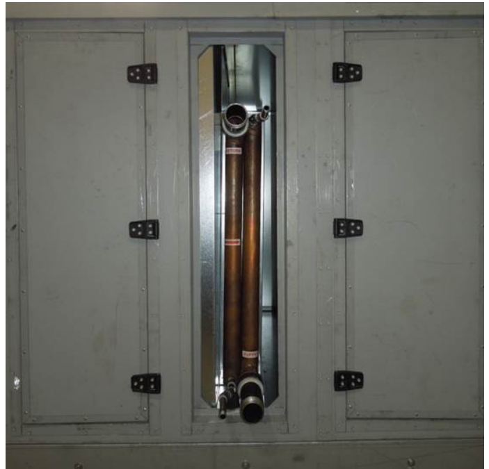
FIGURE 24: UNIT WITH CHILLED WATER COILS ▼
