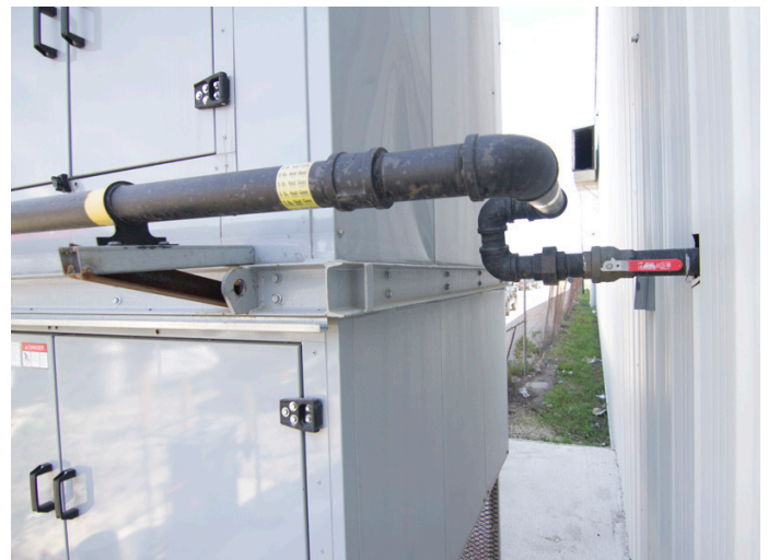
FIGURE 22: TYPICAL GAS LINE SHUT-OFF VALVE ▼
