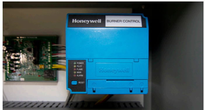
FIGURE 33: FLAME SAFE GUARD CONTROLLER ▼
