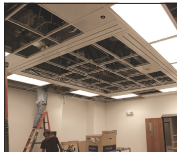
All systems are fully-welded and custom designed for each unique application
